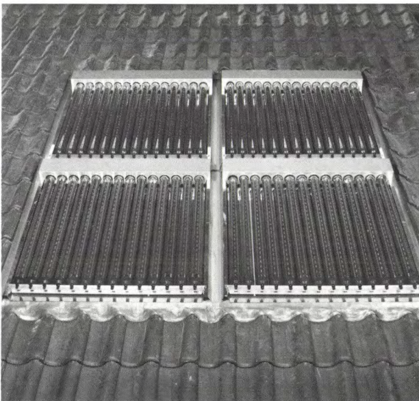
Fig. 19. Four modules with VTR141 tubes, set in a tiled roof.
